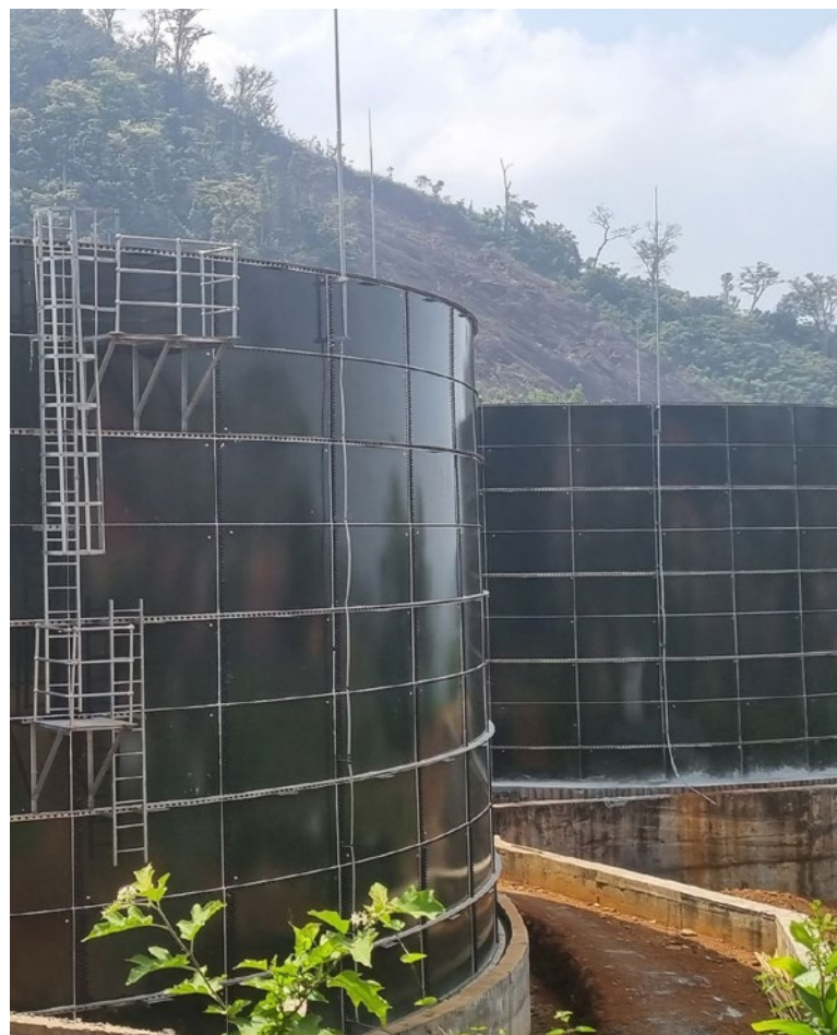
Water tanks from the Freetown WASH and Aquatic Environment Revamping Project, Sierra Leone. Photo by AfDB.
